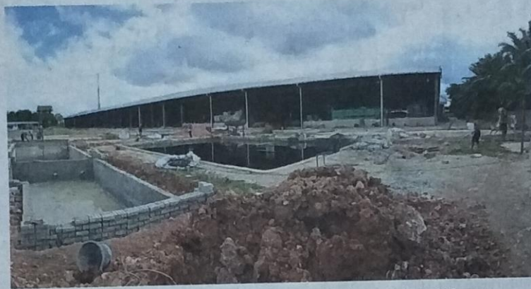
Filtration ponds under construction at the plastic processing factory in Batu 2, Sepang.
